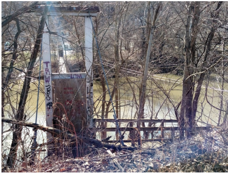
CSX swing bridge over the Jackson River
