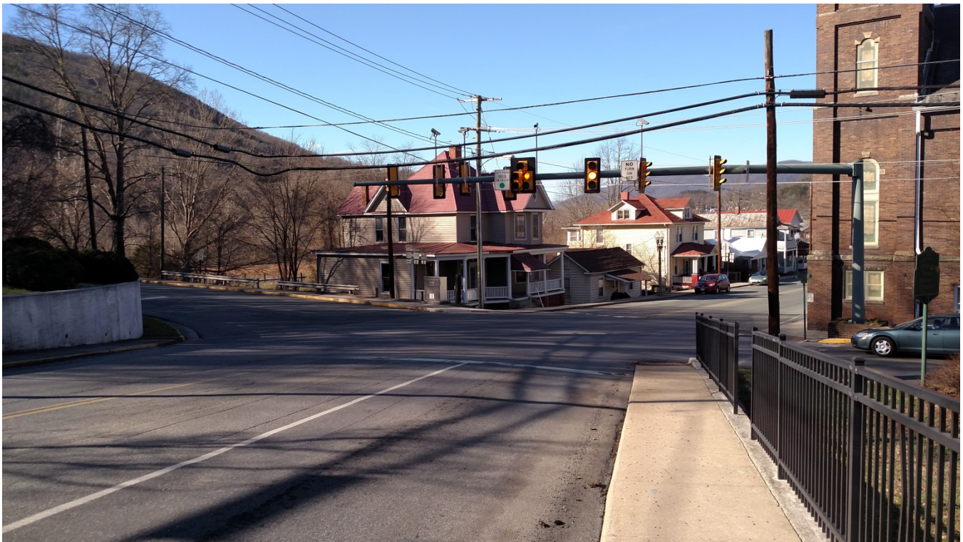
4-way crosswalk markings at Main St & A St lack visibility for approaching vehicles
